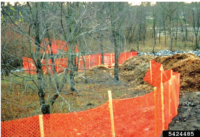
A Vegetation and Soils Protection Zone (VSPZ) around trees, along with woodchip mulch to be used to repair damage to soils post-construction. Credit: Paul Bachi, University of Kentucky Research and Education Center. Creative Commons License 3.0
